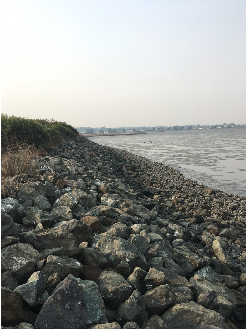
Photograph 5. Outer perimeter of the CRC property (Segment 5). Photograph taken October 10, 2017.
