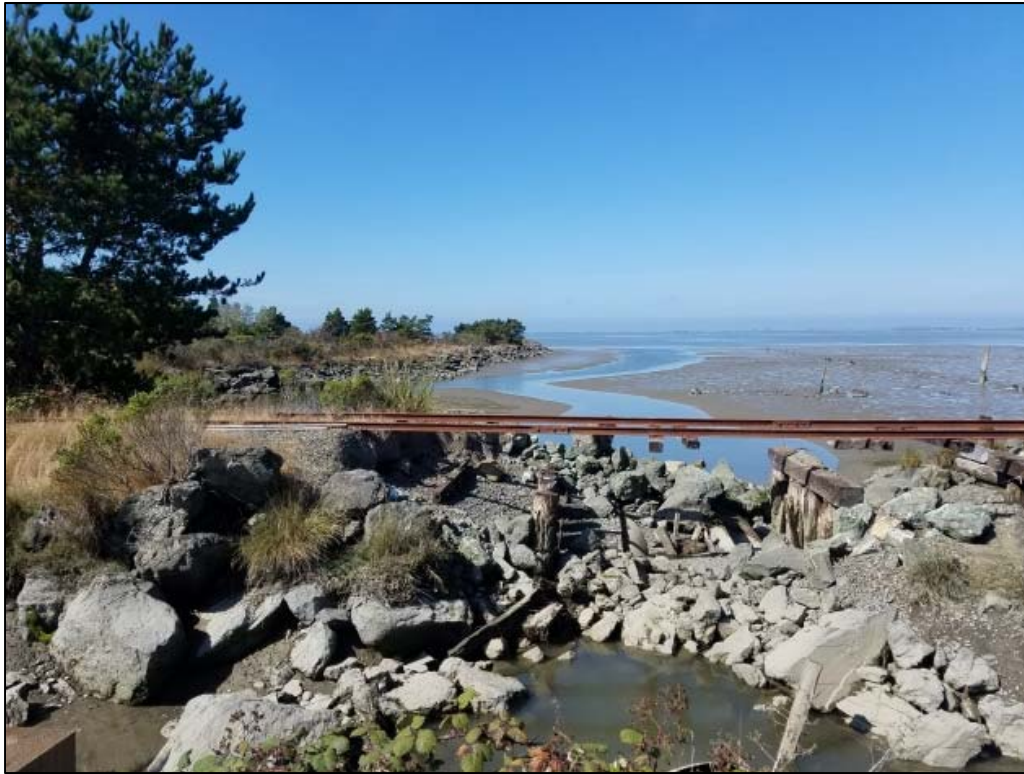
Image 10 (VAU 9, KOP 10). Existing Brainard Slough railroad crossing. View looking west.
