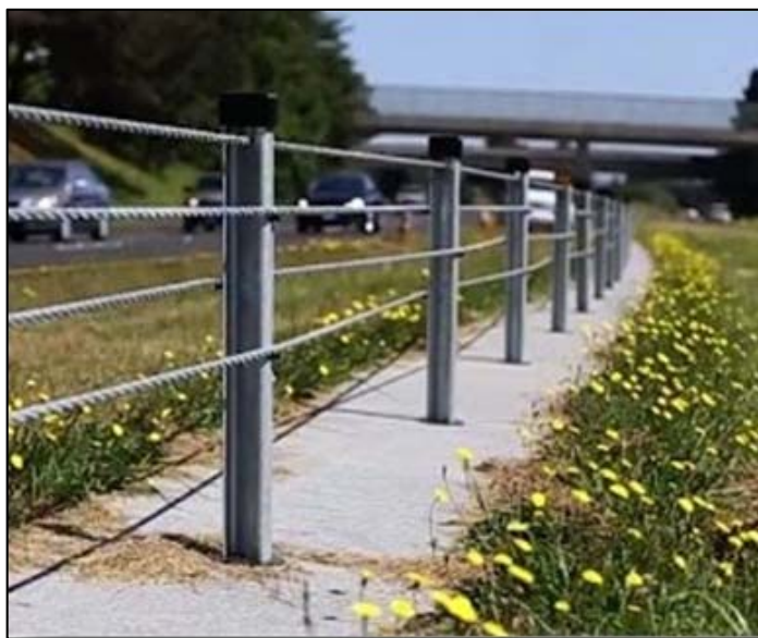
Typical cable barrier fencing (all project segments.)
