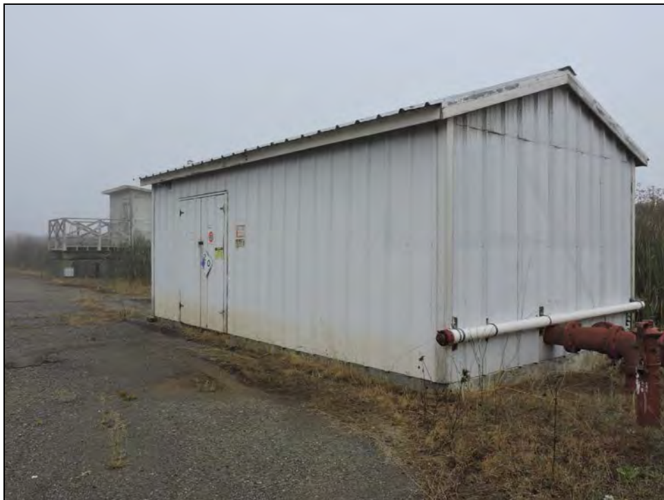
Photograph 11: South and east sides of Building 5 in foreground, Building 6 in background, camera facing northwest, October 25, 2017.
