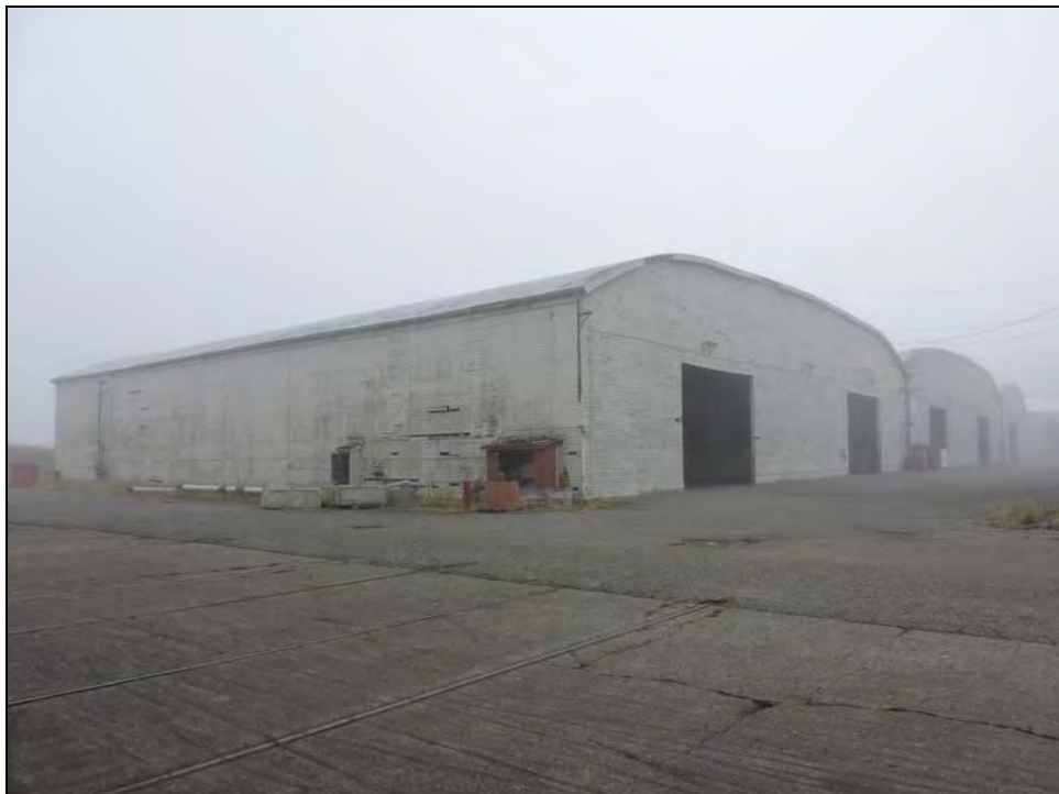
Photograph 9: West and south sides of Building 4, camera facing northeast, October 25, 2017.
