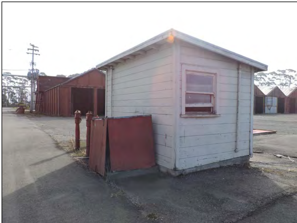
Photograph 17: North and west sides of Building 13, Building 15 in background, camera facing southeast, October 25, 2017.
