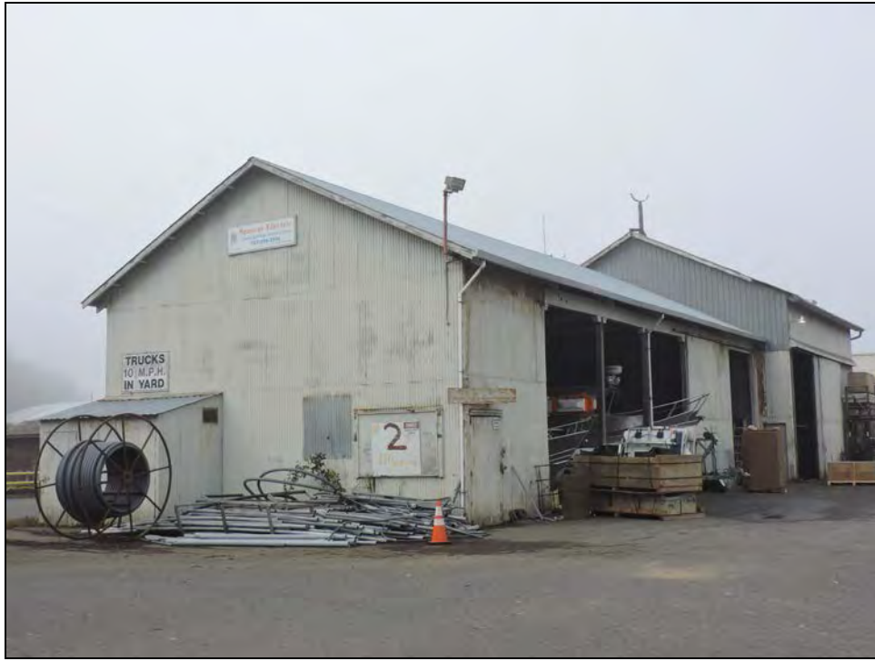
Photograph 32: North and east sides of Building 28, camera facing southwest, October 25, 2017.
