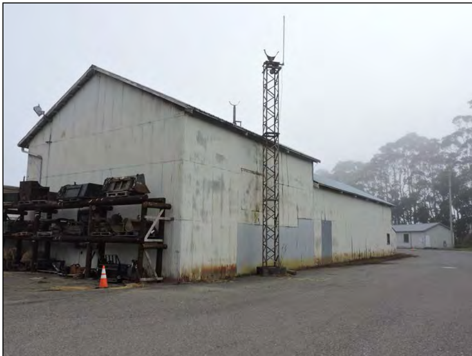
Photograph 33: West and south sides of Building 28, camera facing northeast, October 25, 2017.
