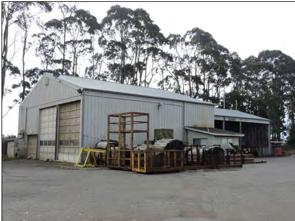
Photograph 23: East and north sides of Building 18, camera facing south, October 25, 2017.
