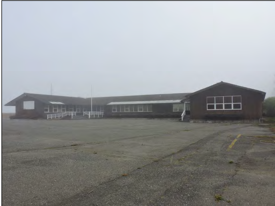
Photograph 2: West side of Building 1, camera facing northeast, October 25, 2017.
