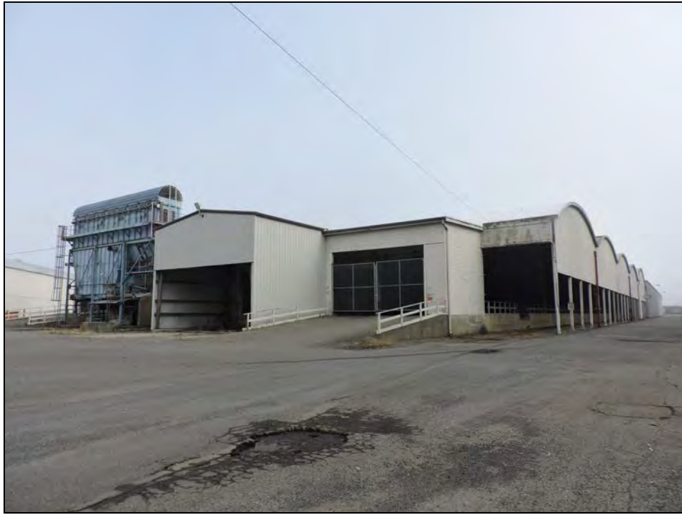
Photograph 8: West end of Building 3, camera facing north, October 25, 2017.
