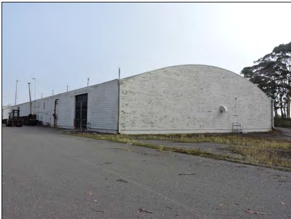
Photograph 25: South and west sides of Building 22, camera facing northeast, October 25, 2017.
