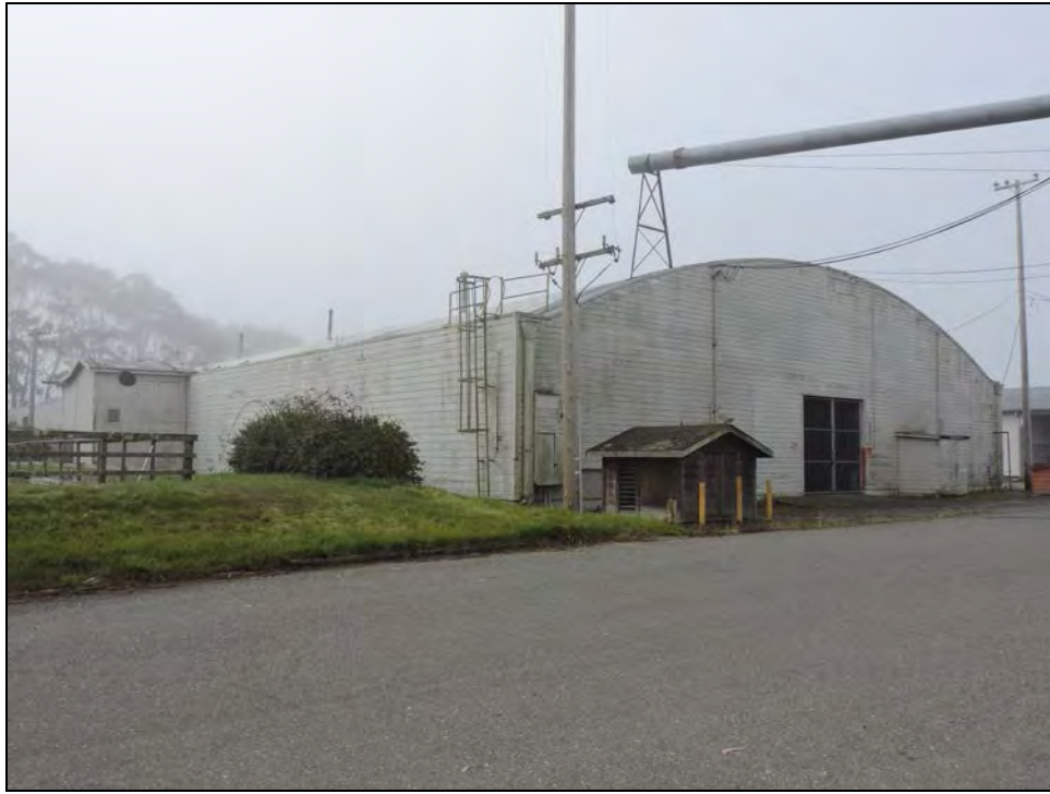
Photograph 26: North and east sides of Building 22, Building 23 in foreground, camera facing southwest October 25, 2017.
