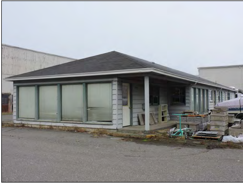
Photograph 30: South and east sides of Building 27, camera facing northwest, October 25, 2017.
