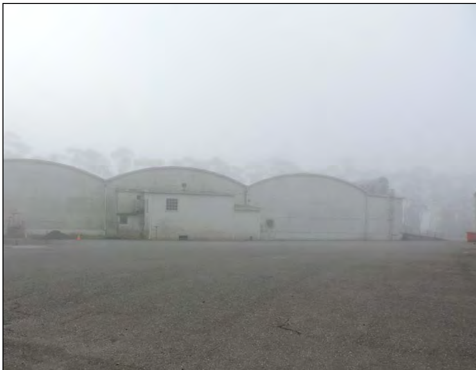
Photograph 7: Two-story shed-roof building section on the north side of the west end of Building 3 (former planing mill), camera facing southeast, October 25, 2017.
