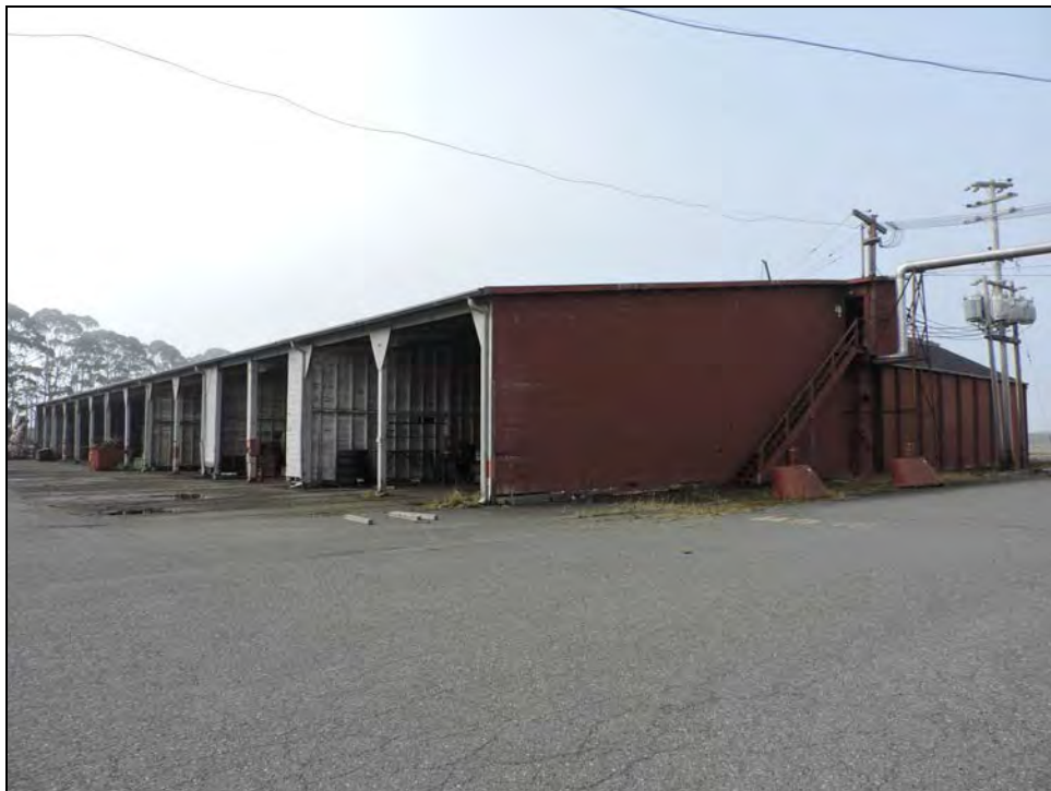
Photograph 21: North and east sides of Building 15, camera facing southwest, October 25, 2017.
