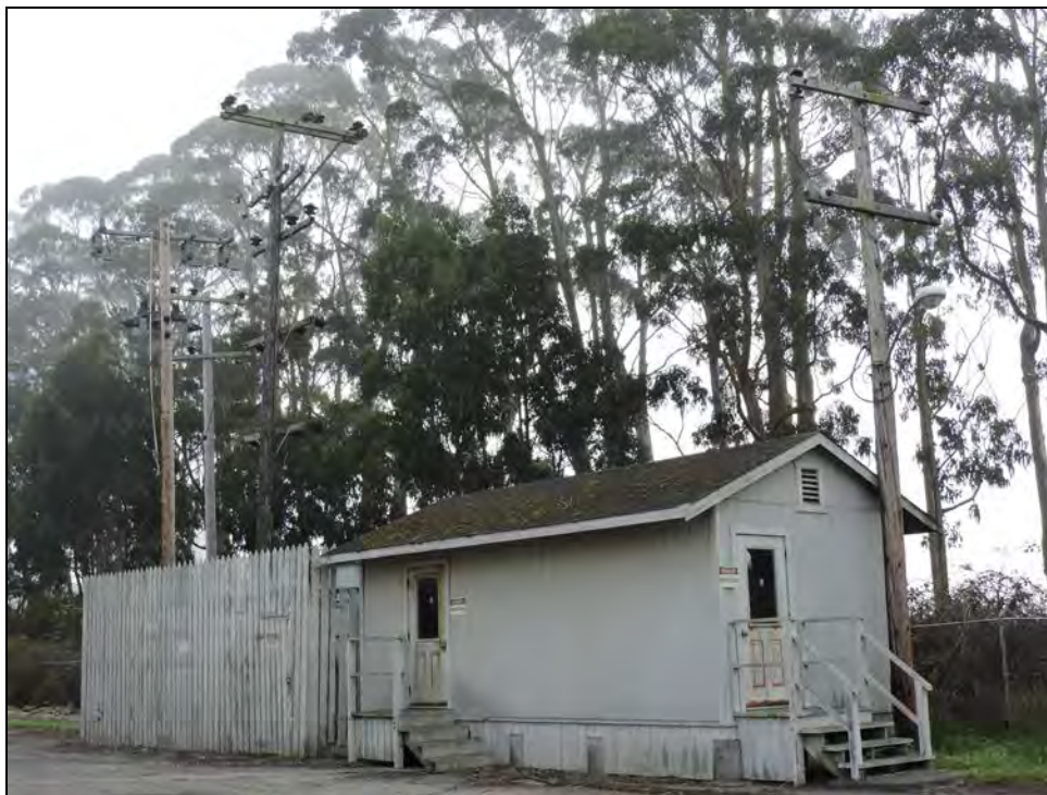
Photograph 37: North and west sides of Building 34, camera facing east, October 25, 2017.
