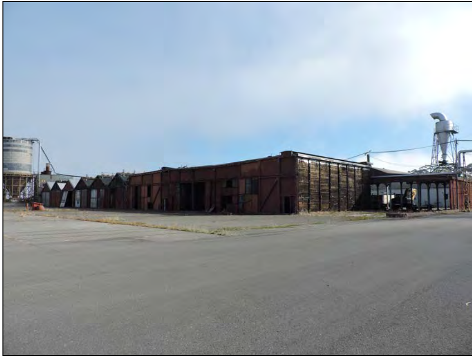
Photograph 18: West and south sides of Building 14, camera facing northeast, October 25, 2017.
