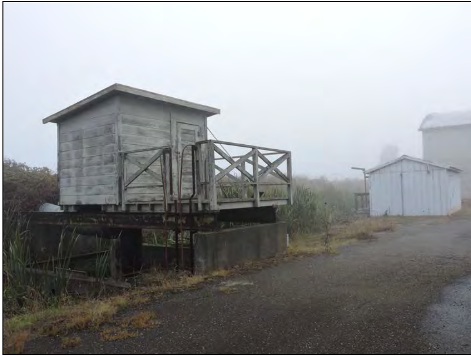
Photograph 12: West and south sides of Building 6 in foreground, Building 5 at right, Building 4 at far right, camera facing northeast, October 25, 2017.
