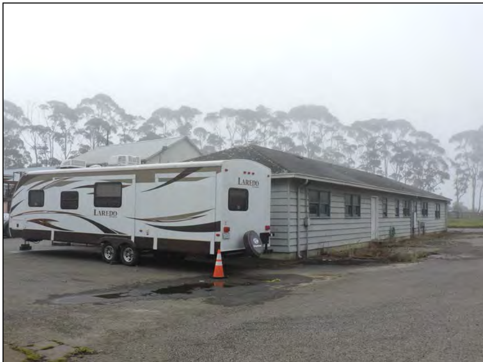
Photograph 31: West and north (obscured) sides of Building 27, camera facing southeast, October 25, 2017.
