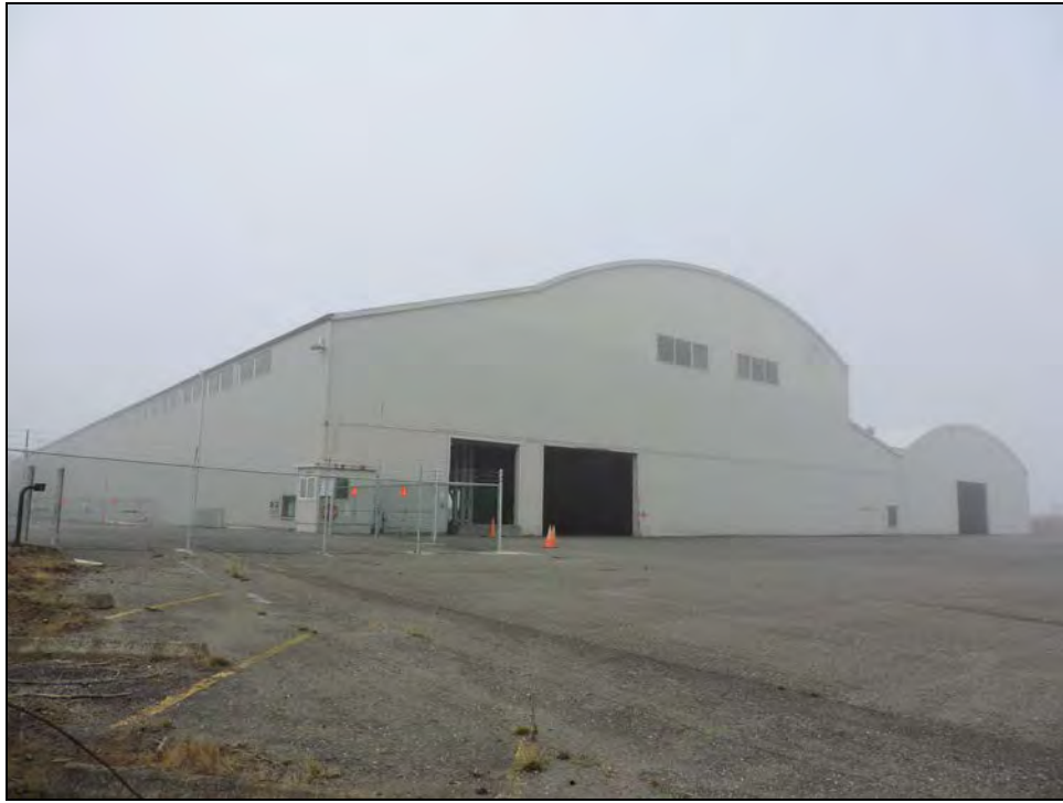
Photograph 4: East and south sides of Building 3, camera facing northwest, October 25, 2017.
