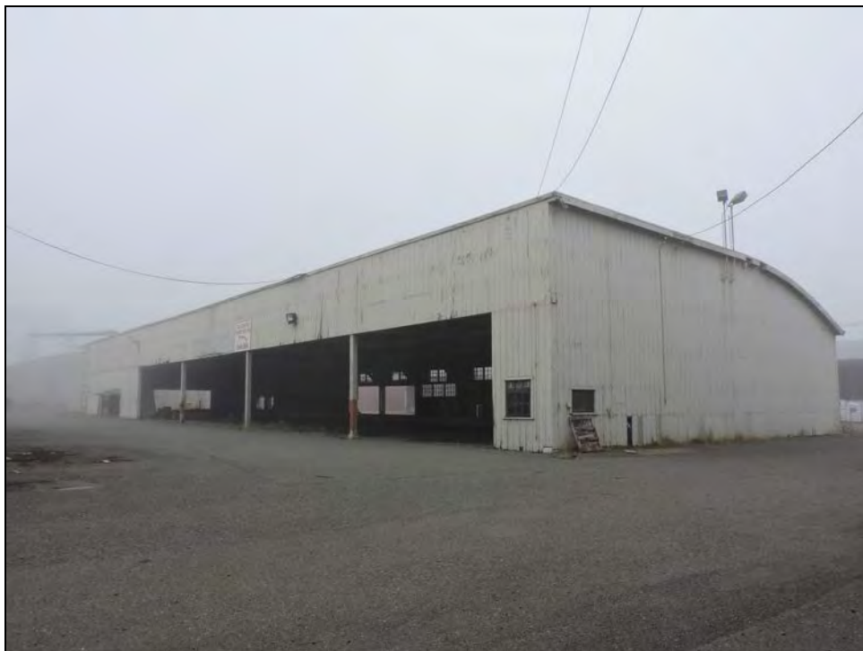
Photograph 27: North and east sides of Building 24, camera facing southwest, October 25, 2017.
