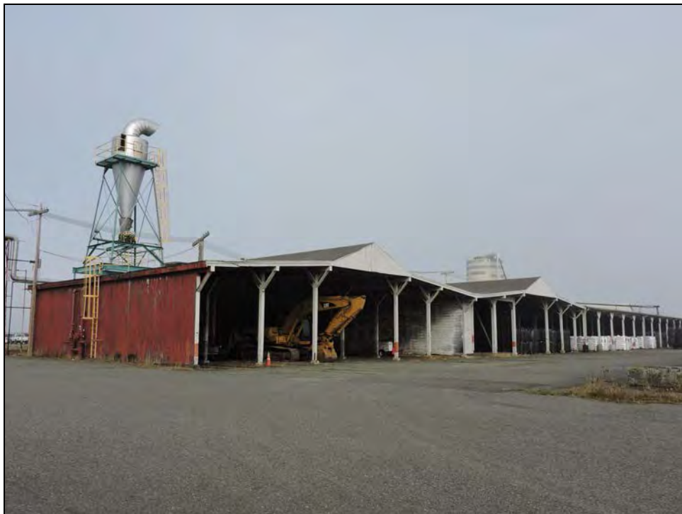
Photograph 19: South and east sides of Building 14, camera facing northwest, October 25, 2017.
