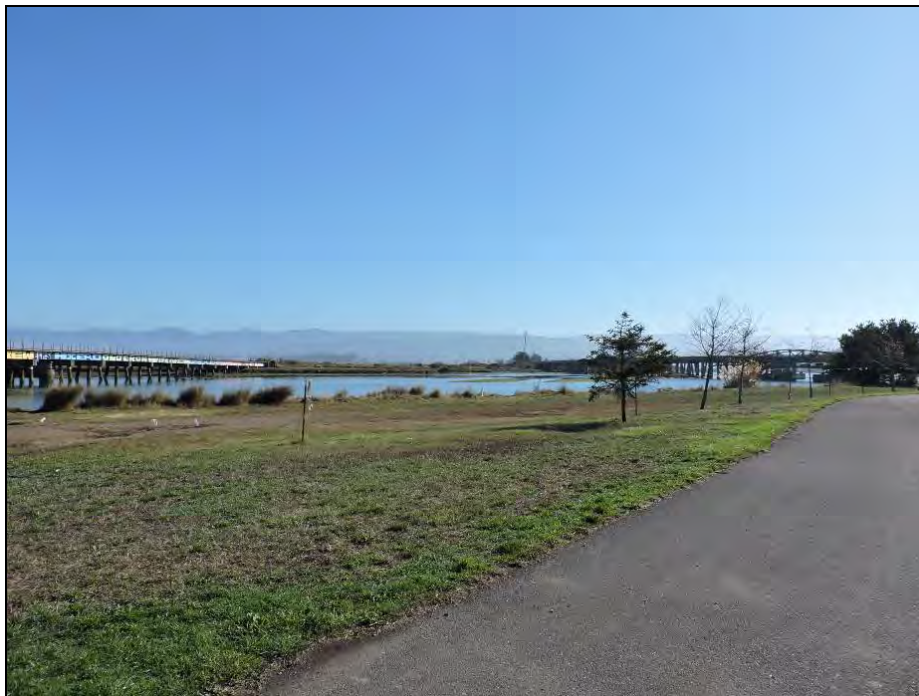
Photograph 6: Eastern approach of modern lift-bridge and elevated track over Eureka Slough in relation to Highway 101, camera facing east, October 25, 2017.
