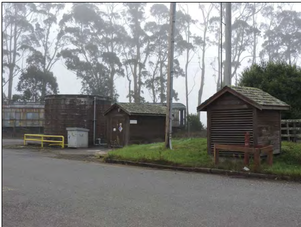
Photograph 35: Building 30 at right, Building 31 at center, and Building 32 at left, camera facing southeast, October 25, 2017.
