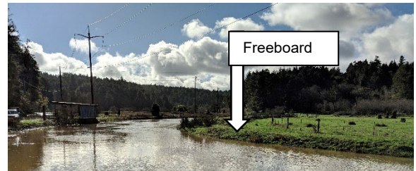
Freeboard between Levee Crest and Tidal Water.
