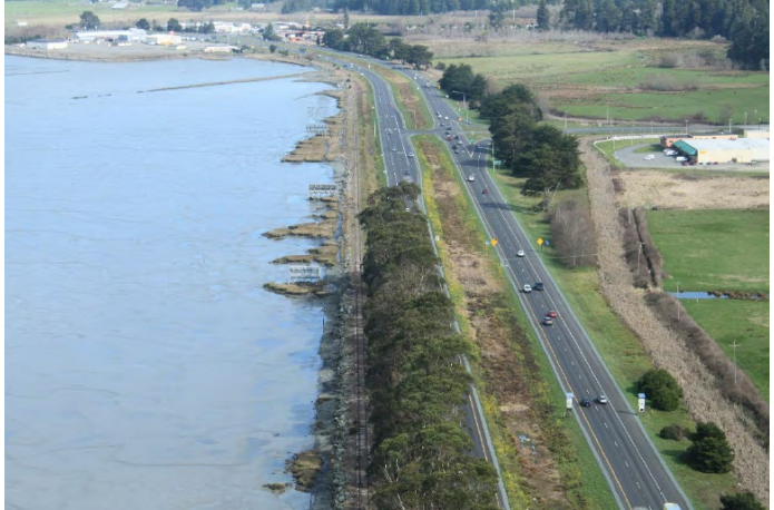
The Planned Humboldt Bay Trail South will Increase the Elevation and Improve Rock Slope Protection Along the Bay Shoreline.
