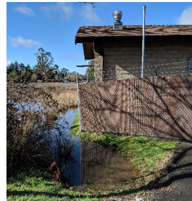
Public Utility Infrastructure within one to two feet of high tides
