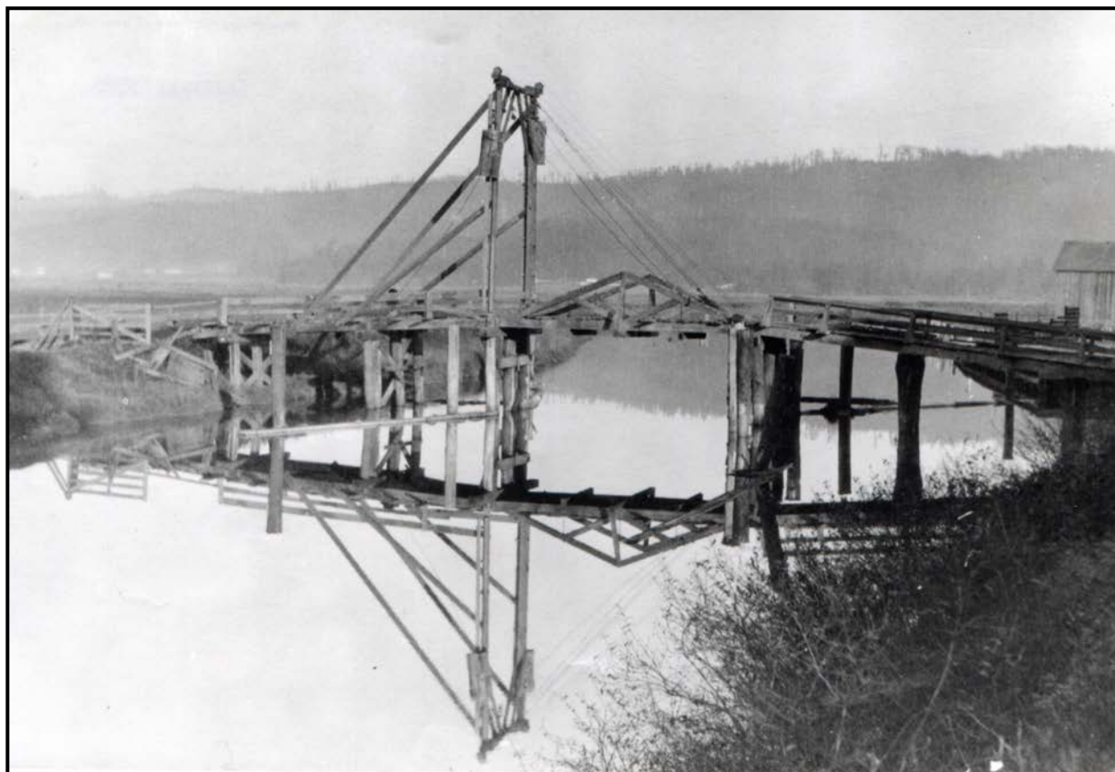
Drawbridge over Freshwater Slough near Myrtle Avenue (HSU Library).
