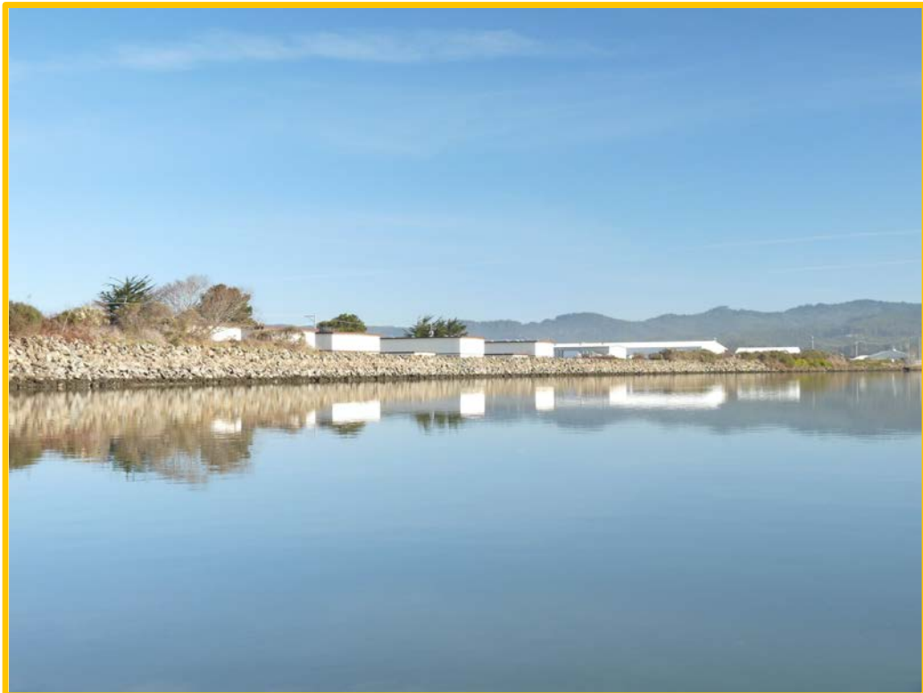
North bank of Eureka Slough, heavily armored (Aldaron Laird).
