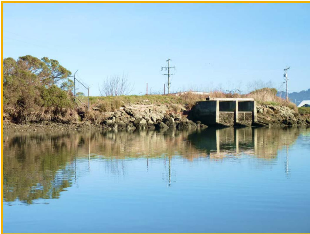
Tide gate near eastern end of Eureka Slough (Aldaron Laird).
