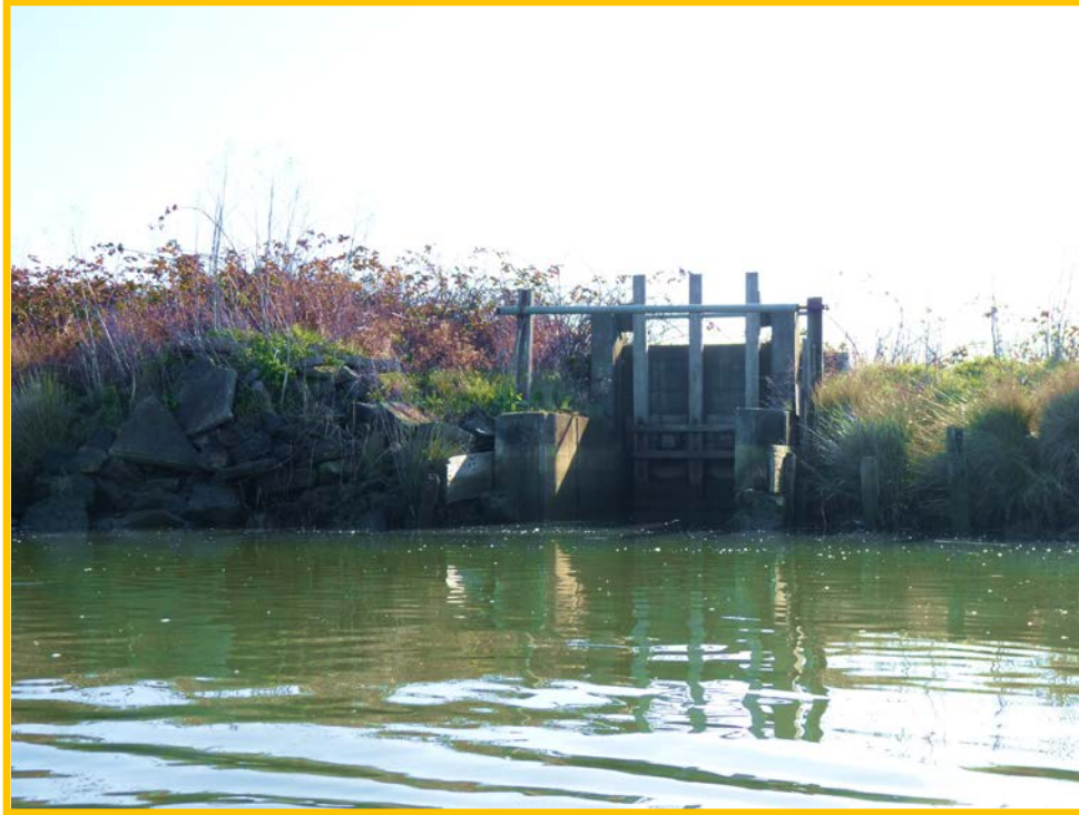
Tide gate on Fay Slough (Aldaron Laird).
