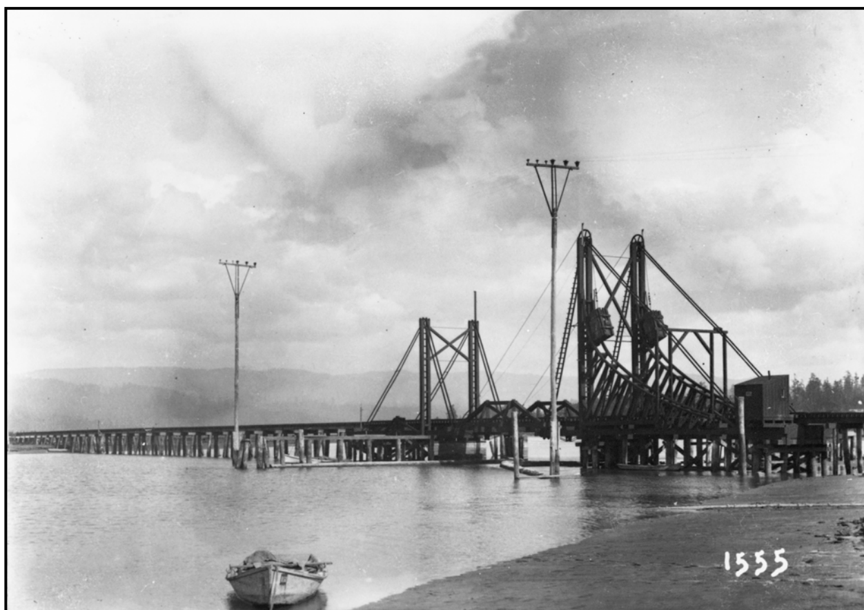
C&N lift bridge over Eureka Slough (HSU Library).
