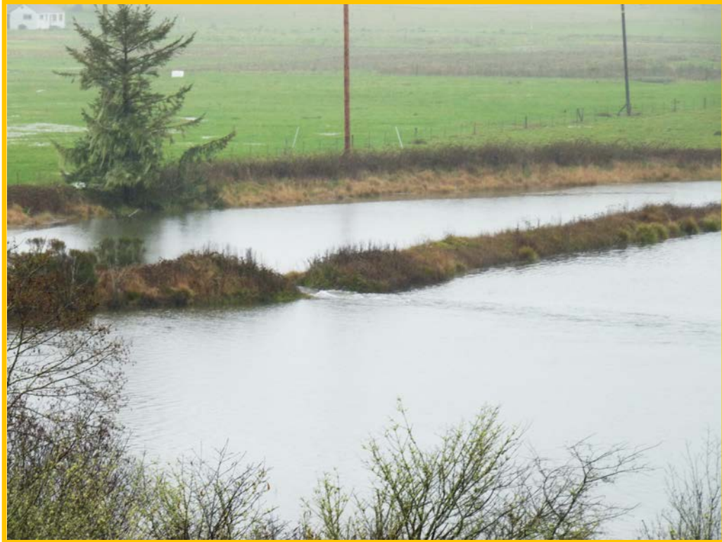
Induced breach of Fay Slough, 2013 (Aldaron Laird).
