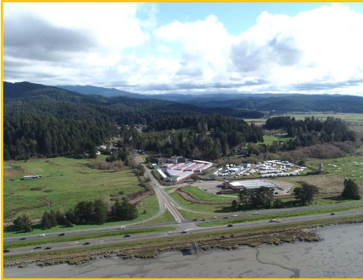
Railbed causeway serving as a dike at Indianola Cutoff (Humboldt County Public Works).
