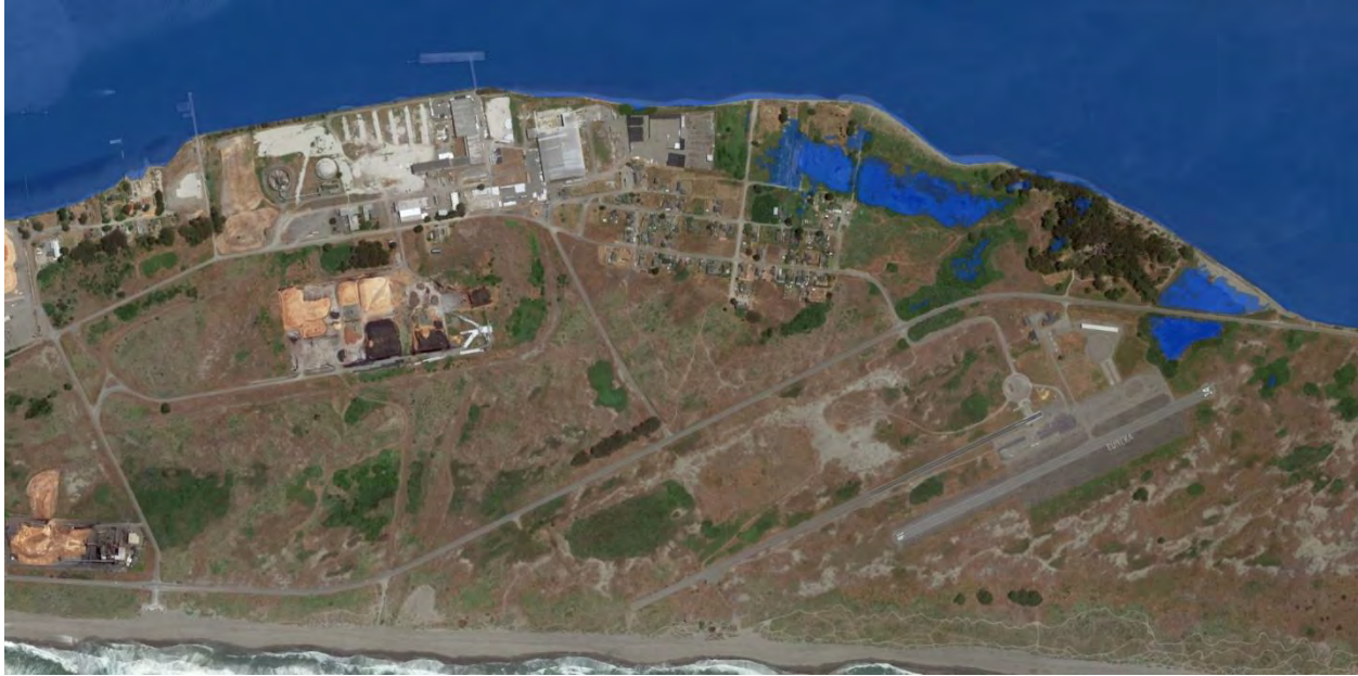
Figure 15. Low-lying wetland areas (blue) that range in elevation from 6 to 9 feet between Fairhaven and the higher elevation dune shoreline of 9 to 10 feet, showing inundation under today's MHHW of 6.5 feet.
