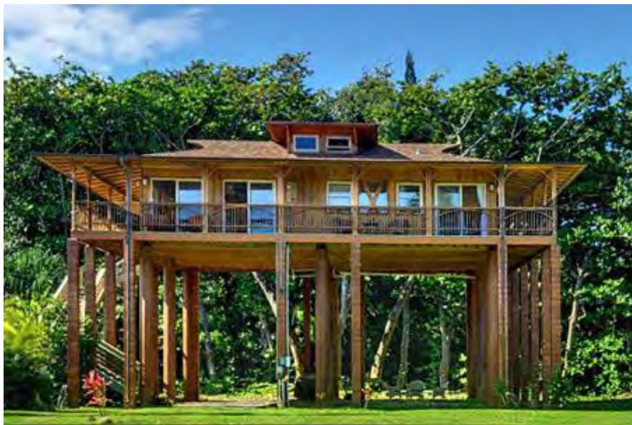
Figure 14. An example of an elevated house in Hawaii with liveable floor area above storm surge elevation.
