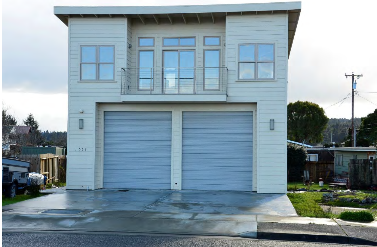
Figure 13. Example of a residential structure with a break-away first story and livable second story, recently construction in King Salmon.
