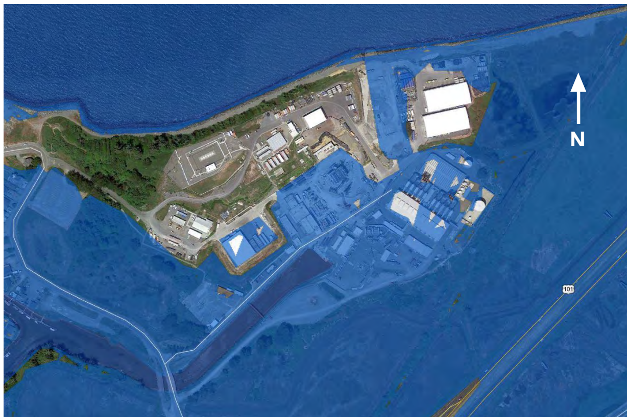
Figure 7. Tidal inundation of King Salmon Avenue, PG&E's Humboldt Bay Generating Station, former Humboldt Bay Power Plant, two access roads, and a portion of the sea wall on Humboldt Bay during MAMW or king tides with 3.3 feet (1.0 meter) of sea level rise (9.8 feet NAVD 88) by 2065, based on a high projection (OPC 2018), assuming shoreline barrier structures do not exist or are breached.
