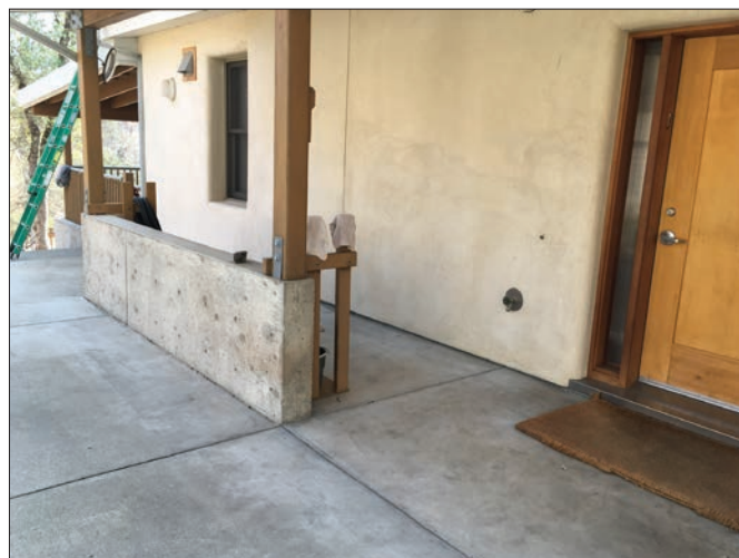
The vertical and horizontal noncombustible zone helped this house survive the 2018 Carr Fire.
