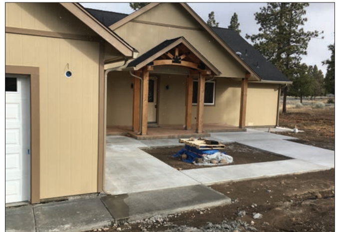
The combination of defensible space and hardening will provide your house the best chance of surviving a wildfire. This newly constructed home utilized fire resistant construction materials and incorporated an essential noncombustible zone.
