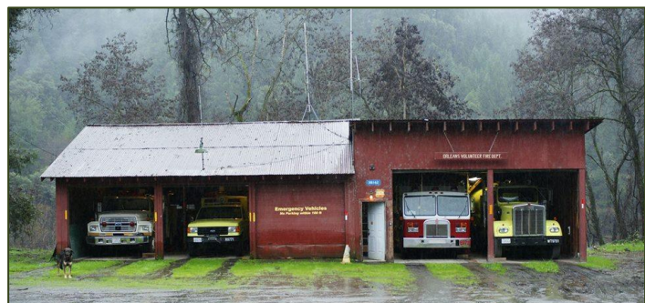
Orleans Fire Engine Bay. Photo: OVFD.
