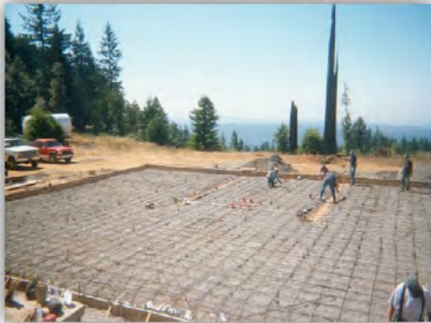
Firehouse Foundation Construction.
