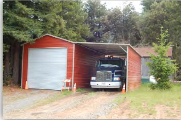
Current Fire Station, Lindsay Green, May, 2015.
