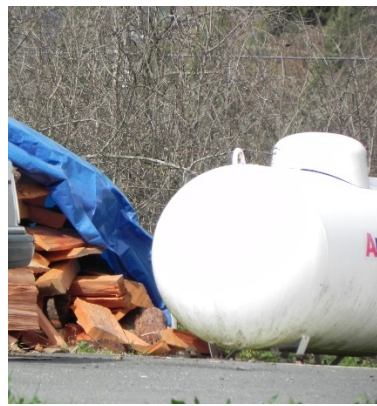
Figure 14: Examples of residential fire risk in high density communities on the Hoopa Valley Indian Reservation. A) Firewood stacked next to house and B) Firewood stacked next to propane tank
