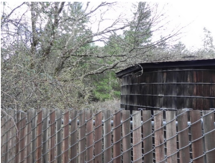
Figure 11: Picture showing vegetation including Himalayan Blackberry encroachment on water tank.
