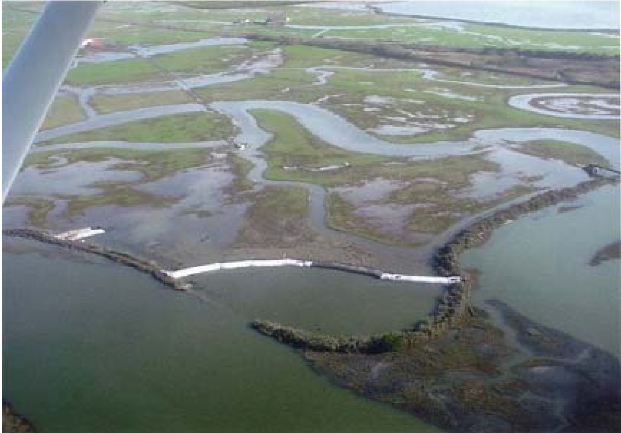
Figure 15.. An earthen dike breached during king tide and high waves in 2003 resulted in hundreds of acres flooded by saltwater, with a temporary water cofferdam (Times-Standard Andrew Bird photograph January 26, 2004).
