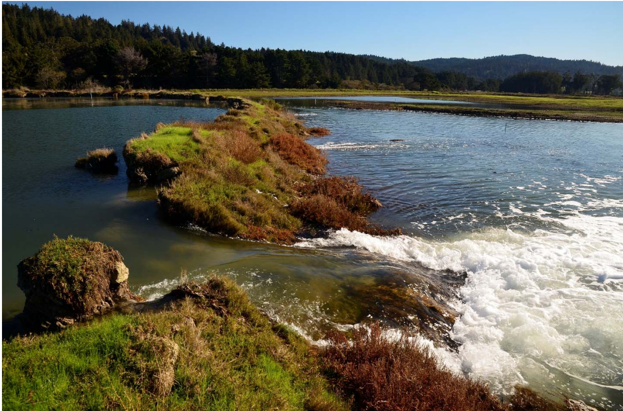
Figure 6. Dike breaching during a king tide, inundating low-lying former tide lands.
