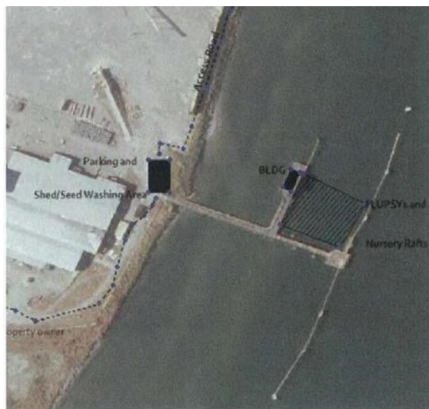
Figure 4-19: Taylor Mariculture Co Facilities in Humboldt Bay
