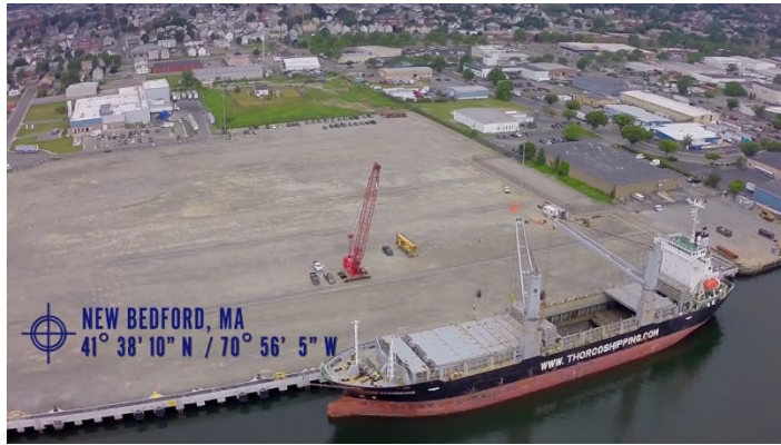
Figure 2: New Bedford Marine Commerce Terminal
