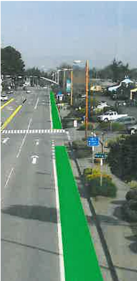
Central Avenue in McKinleyville features improved, green bicycle lanes.
