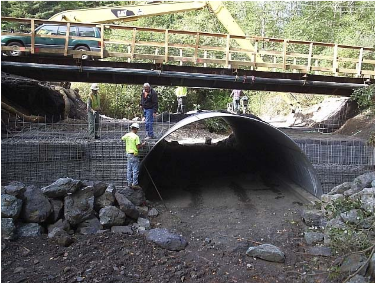
Public Works' fish-friendly culvert replacement project at Grassy Creek.
