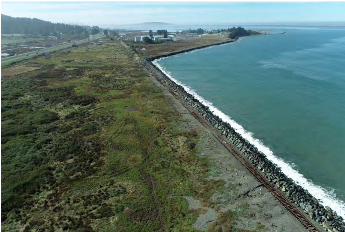
Image 7: View facing south of Segments 1 and 2.
