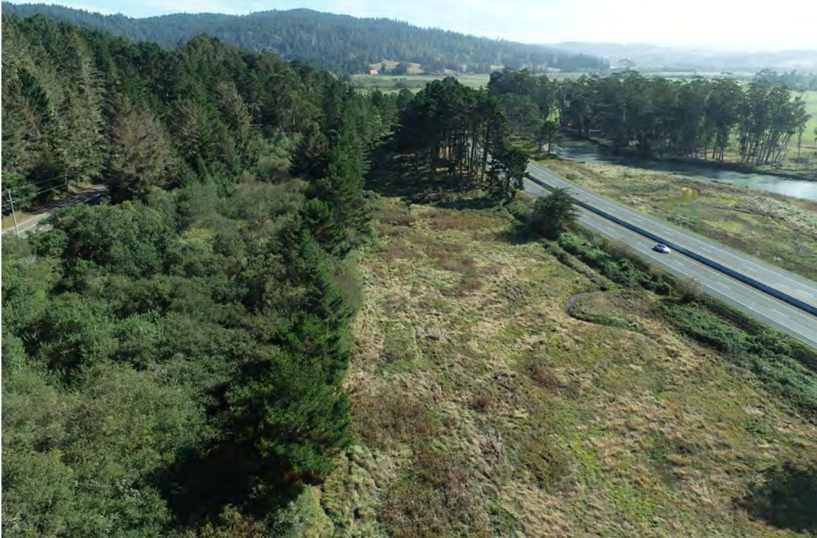
Image 19: Railroad corridor between Highway 101 and Tompkins Hill Road (Segment 4).
