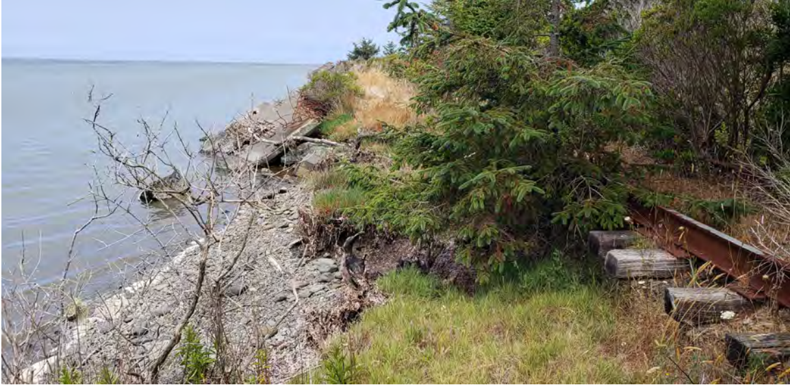
Image 17: Shoreline erosion and concrete rubble (Segment 3).
