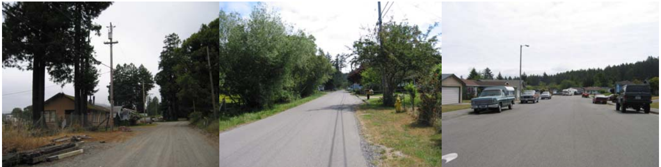
Residential streets vary greatly throughout Humboldt County. From left to right, an unpaved rural road in Carlotta, paved road with swale in Fortuna, and a larger road with sidewalks in Eureka/Humboldt Hill.
