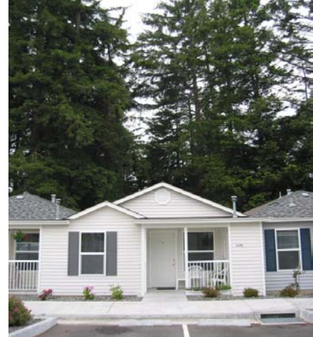
Front porches and walkways can create a pedestrian-friendly environment.
