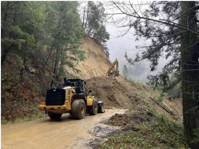
Humboldt County Public Works roads crews work to repair a slide on Seely McIntosh Road in February 2025.
