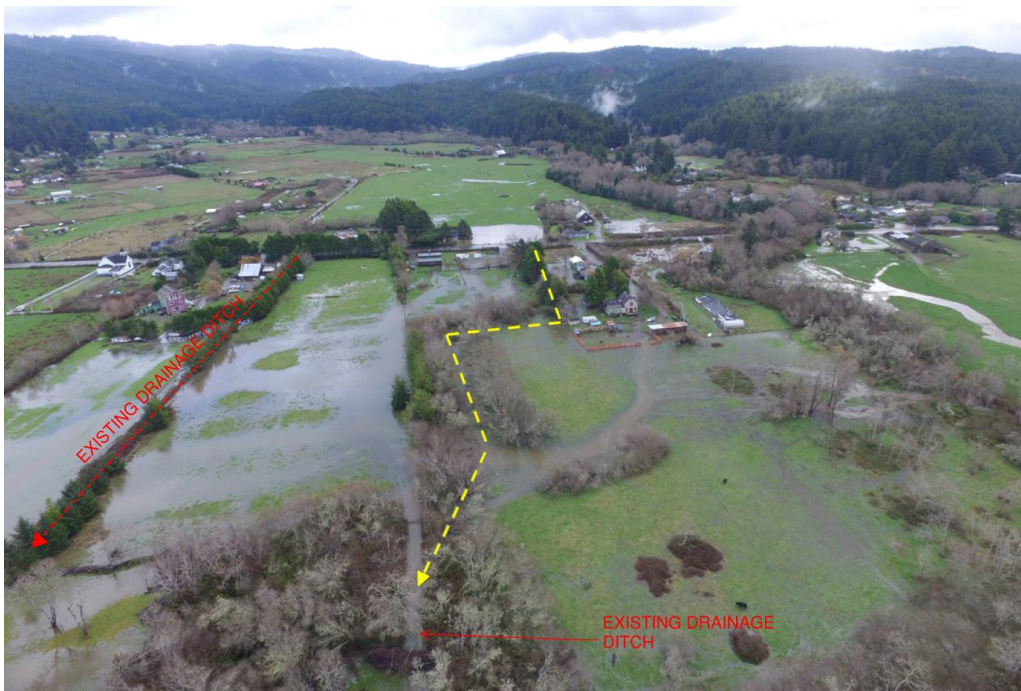
Figure 6 Existing drainage ditch on APN 50106112, proposed drainage ditch, and existing drainage ditch on APN 50106118 / APN 50106112. The dashed yellow line represents the proposed drainage ditch. The drainage ditch will carry shallow concentrated flow to the head of the arrow, where the drainage ditch will terminate.
