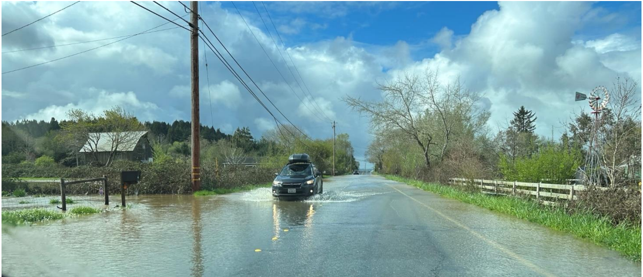
Figure 3 Flooding on OAR (looking south)
