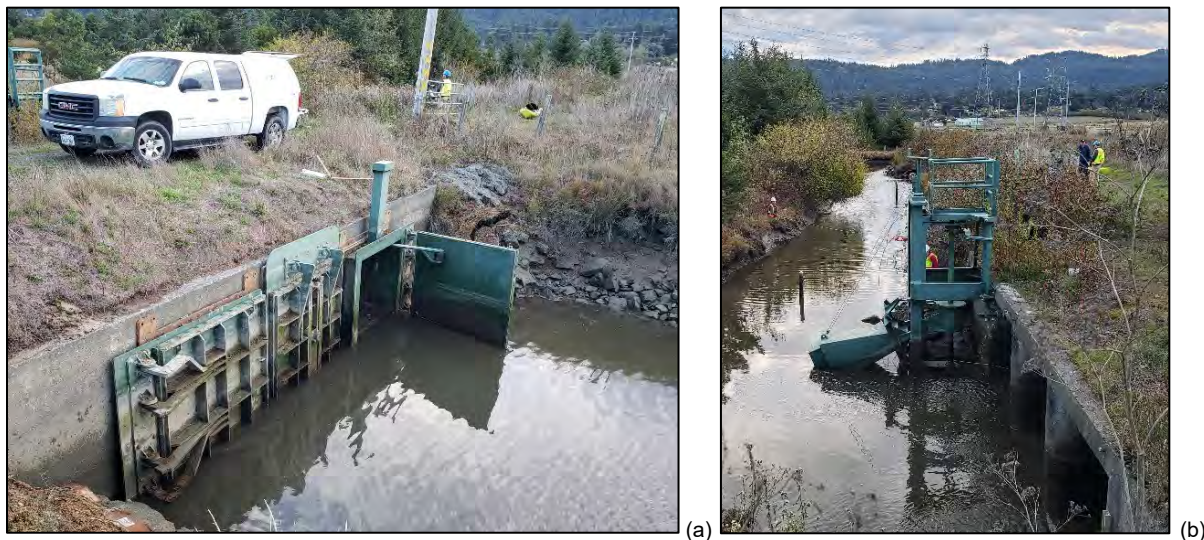
Figure 2-8. The Caltrans maintained Gannon Slough (a) tide gates and (b) MTR float.
