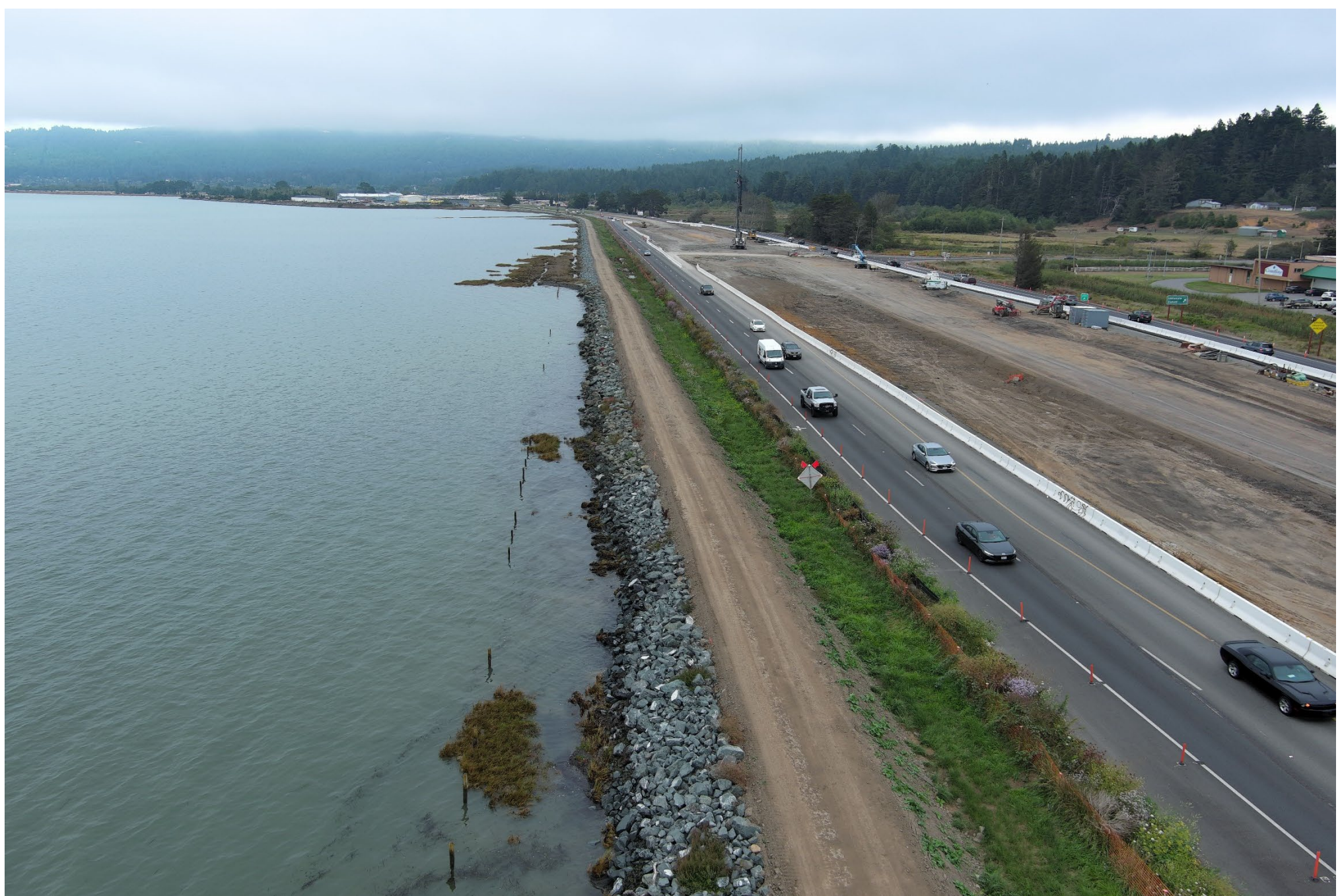
Humboldt Bay Trail construction in progress
