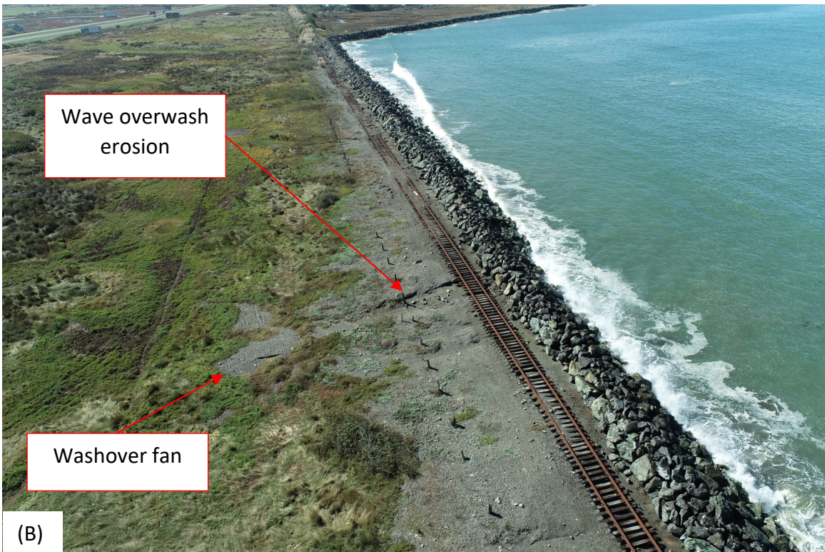
Figure 9. 2023 oblique aerial view of Shoreline Reach 1 existing rock revetment and dislodged rock along beach and on top of railroad grade (A); and localized overwash erosion and washover fan of the railroad grade fill from wave runup and overtopping behind the revetment (B). Drone images provided by County of Humboldt.
