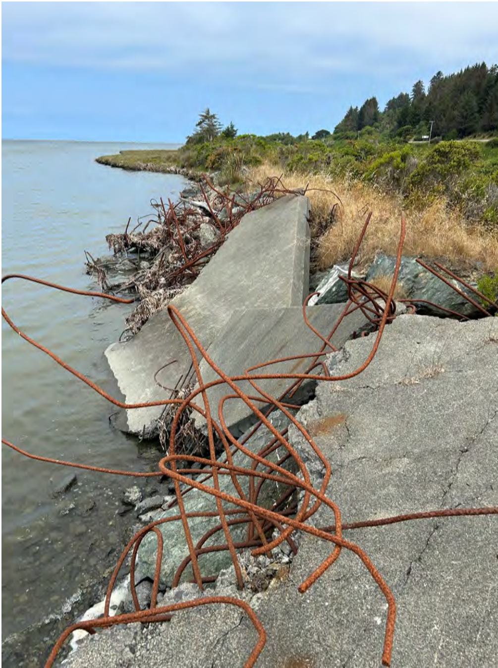
Photo 7. Concrete riprap on the shore of Humboldt Bay south of Fields Landing.
