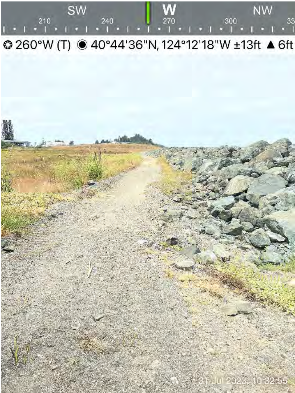
Photo 4. PG&E access corridor north of the Humboldt Bay Power Station, adjacent to the seawall.
