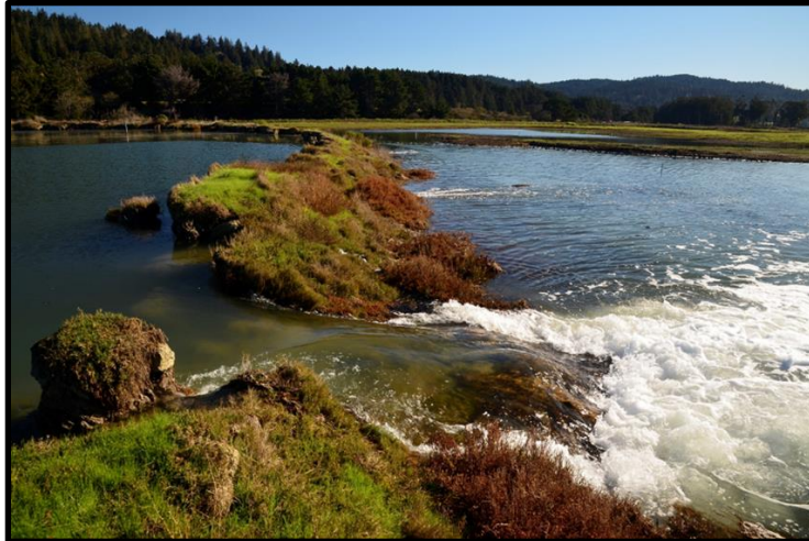
Overtopped dike in low-lying former tidelands of Humboldt Bay following King tides in 2018. Photo credit to Aldaron Laird.
