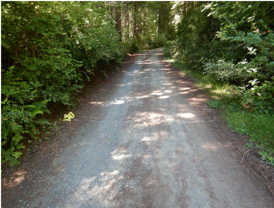
Portion of R-1 road (May 25, 2022)
