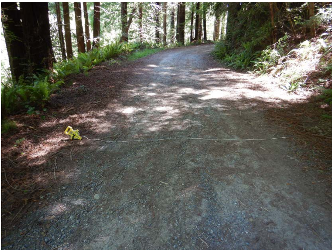
Portion of R-1 road (May 25, 2022)
