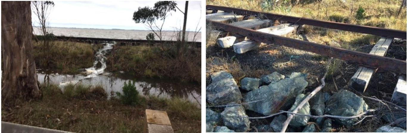
Figure 4 Rail prism erosion and tidal overtopping in project area. Photo source, HCDPW.
