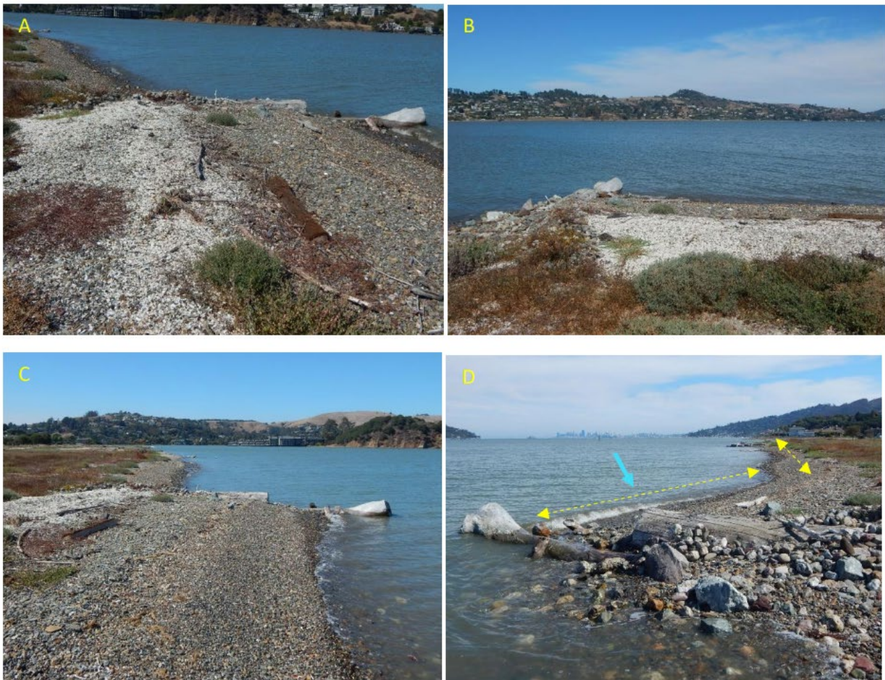
Figure 62 Example photos of gravel beach with groins or drift sills of embedded, pinned logs along the Aramburu Island project shoreline in North San Francisco Bay used to trap updrift coarse sediment (A-C). Downdrift side of groins either remain stable or exhibit erosion where the drift beach sediment is obstructed locally (B-D). When gravel beach profiles retreat landward overtime, beach accretion on the updrift side reorient to face dominant wave approach (blue arrow), in contrast with the strongly oblique orientation of the main beach axis relative to the wave approach (SFEI 2020).
