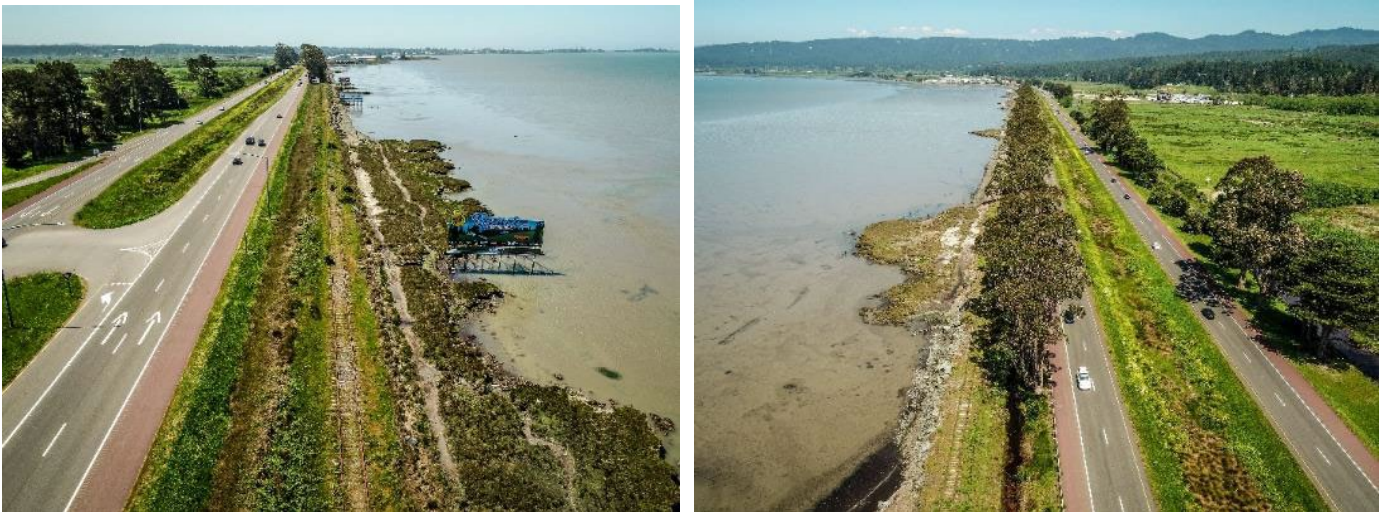
Figure 1 Project shoreline between Brainard and Bracut showing Highway 101, rail prism and variable intertidal shoreline conditions facing south at Indianola Interchange (left) and north (right). Photo source, HCDPW.
