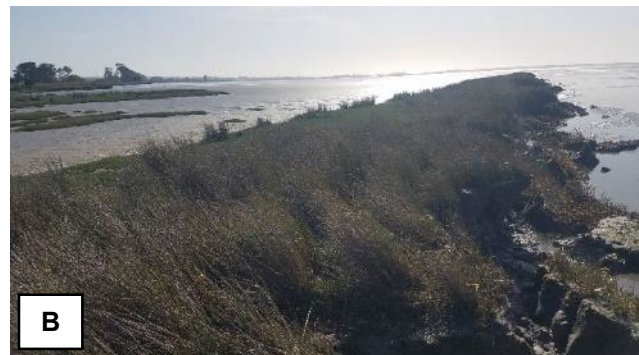
Oblique Photo 1: (A) Salt marsh scarp with thin (1-2 inch) fine sand deposit on adjacent mudflat. (B) Scarping with Spartina dominated failure blocks on windward (north) side of constructed remanent levee and pickleweed dominated low marsh on lee (south) side.
