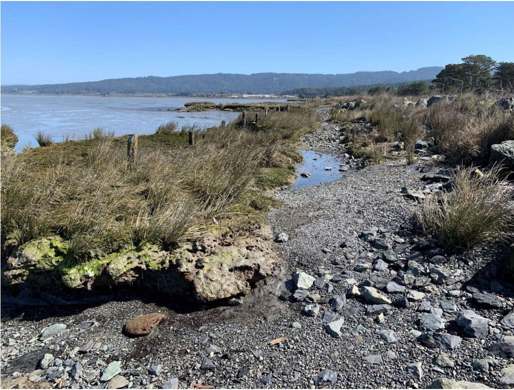
Photo 5. Eroding fringe salt marsh.
