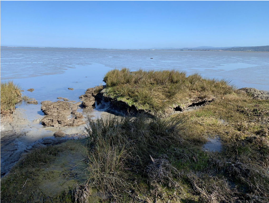
Photo 3. Undercut eroding salt marsh at low tide.
