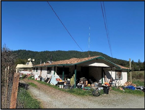
Photos of Salmon Creek Dwellings Examples of the various levels of home hardened dwellings.
