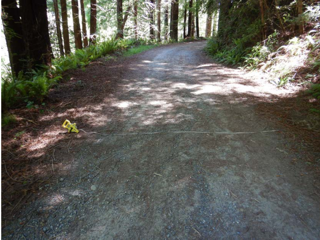
View of portion of R-1 road (May 25, 2022)
