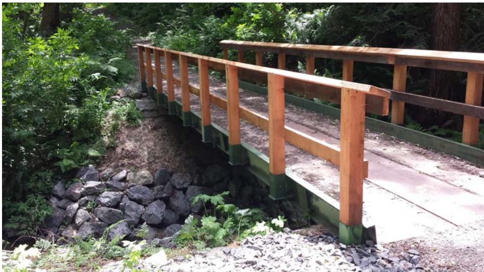
Photo 4-3: Railcar Bridge, Arcata Ridge Trail
