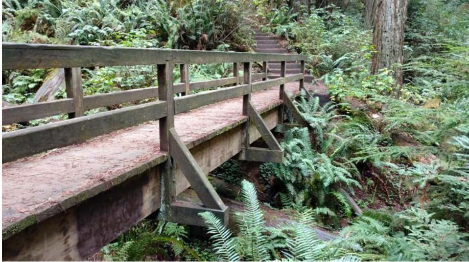
Photo 4-1: Wood Bridge, Arcata Community Forest
