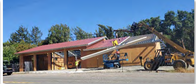
New Briceland Fire Station Under Construction
