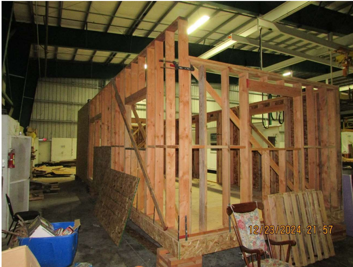
Photo of Home #2 Under Construction in the Hoopa Modular Plant:
